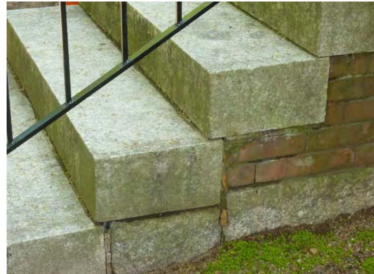
Repair and caulking at granite stairs in Year 1.
