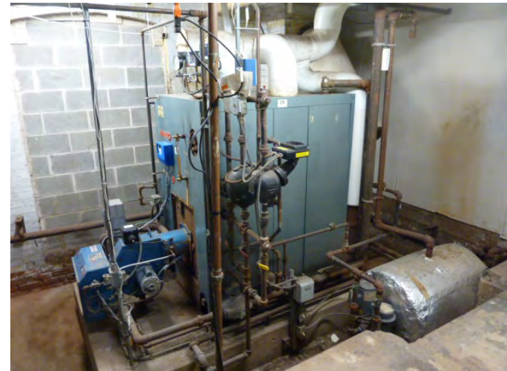
Gas fired heating water boiler is shown to be replaced in Year 3.
