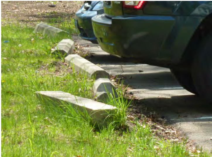
Curb stops to be reset and pinned.
