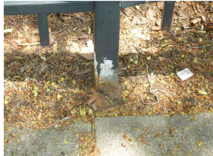
Typical rusted post at ornamental aluminum fence scheduled to be replaced.
