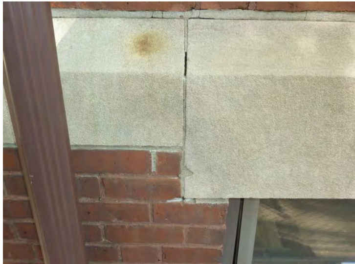
Cracked and open grout joints at the concrete trim on the brick facades are scheduled to be repaired.
