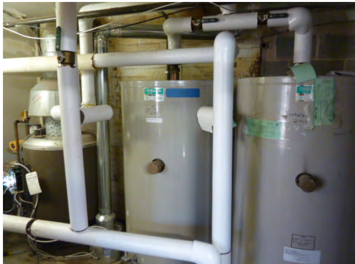
Gas fired domestic hot water heater and storage tanks shown to be replaced in Year 3.
