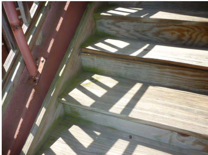
Wood tread nosings are cracked and shearing off, creating trip hazards. Repairs at egress stairs are shown in Year 1.
