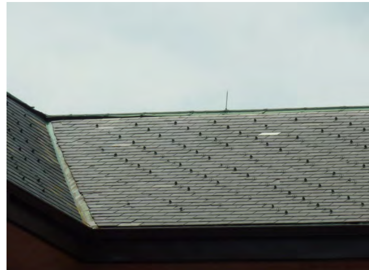
Patches indicate slate shingle replacements. Regular maintenance and repairs are shown over the plan.
